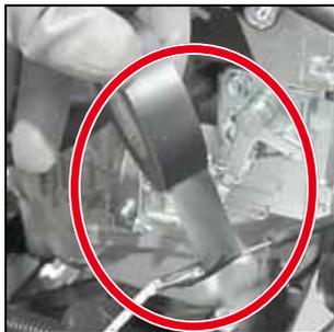
of the old cable to a cable or a cable pulling probe, using a sufficiently strong and reliable adhesive tape.
